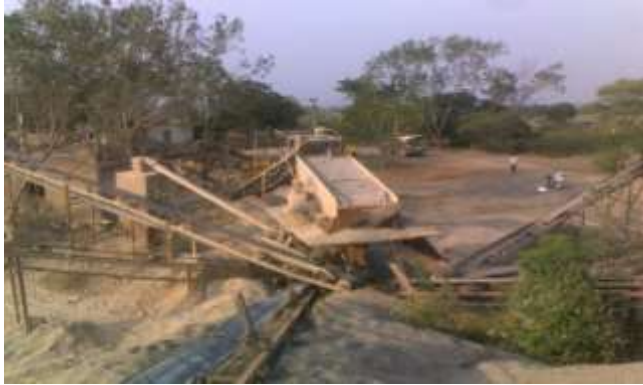
Fig 6: Crushing of Lime stone Aggregate in crusher.
