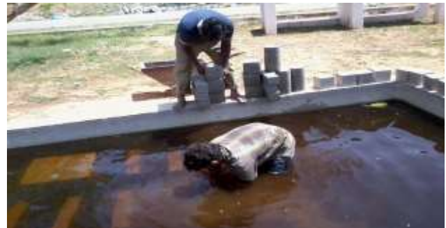
Fig 8: View of the Specimens cured in the Water Tank
