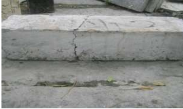
Fig 16: Tested specimens of beam (a)
